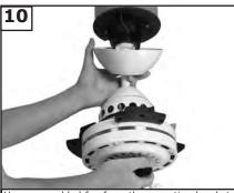
Hang assembled fan from the mounting bracket installed to ceiling in previous step. Make sure the fan is hanging straight. Rotate fan until the tab on the Mounting bracket engages the slot on the Downrod Ball. This must be done to prevent the fan body from rotating when the blades are in motion.
